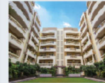
SHALIMAR DWELLING AP SEN ROAD LUCKNOW
