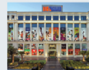
SHALIMAR ELLDEE PLAZA BHOOTNATH MARKET LUCKNOW
