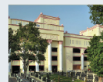
MULTILEVEL PARKING HAZRATGANJ LUCKNOW
