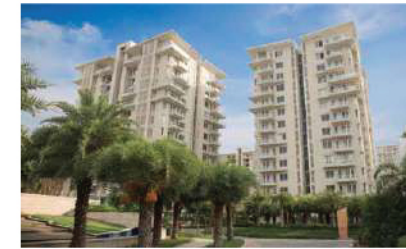
Shalimar Gallant, Mahanagar, Lucknow, UPRERAPRJ3168
