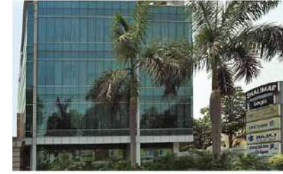
Shalimar Logix, Rana Pratap Marg, Lucknow
