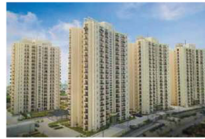
Vista, Gomti Nagar Extension, Lucknow, UPRERAPRJ4833
