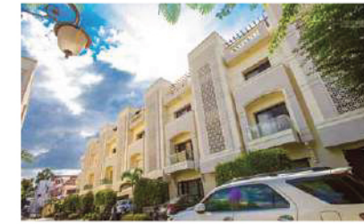
Shalimar Meadows, Gokhale Marg, Lucknow
