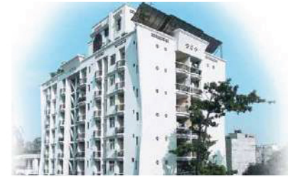
Shalimar Apartments, P. N Road, Lucknow
