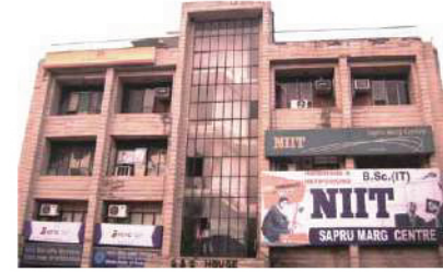
SAS House, Sapru Marg, Lucknow
